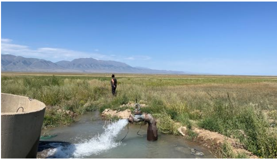
Figure 5 The pipe connected to the central system. Photo by naMec, 2024.
